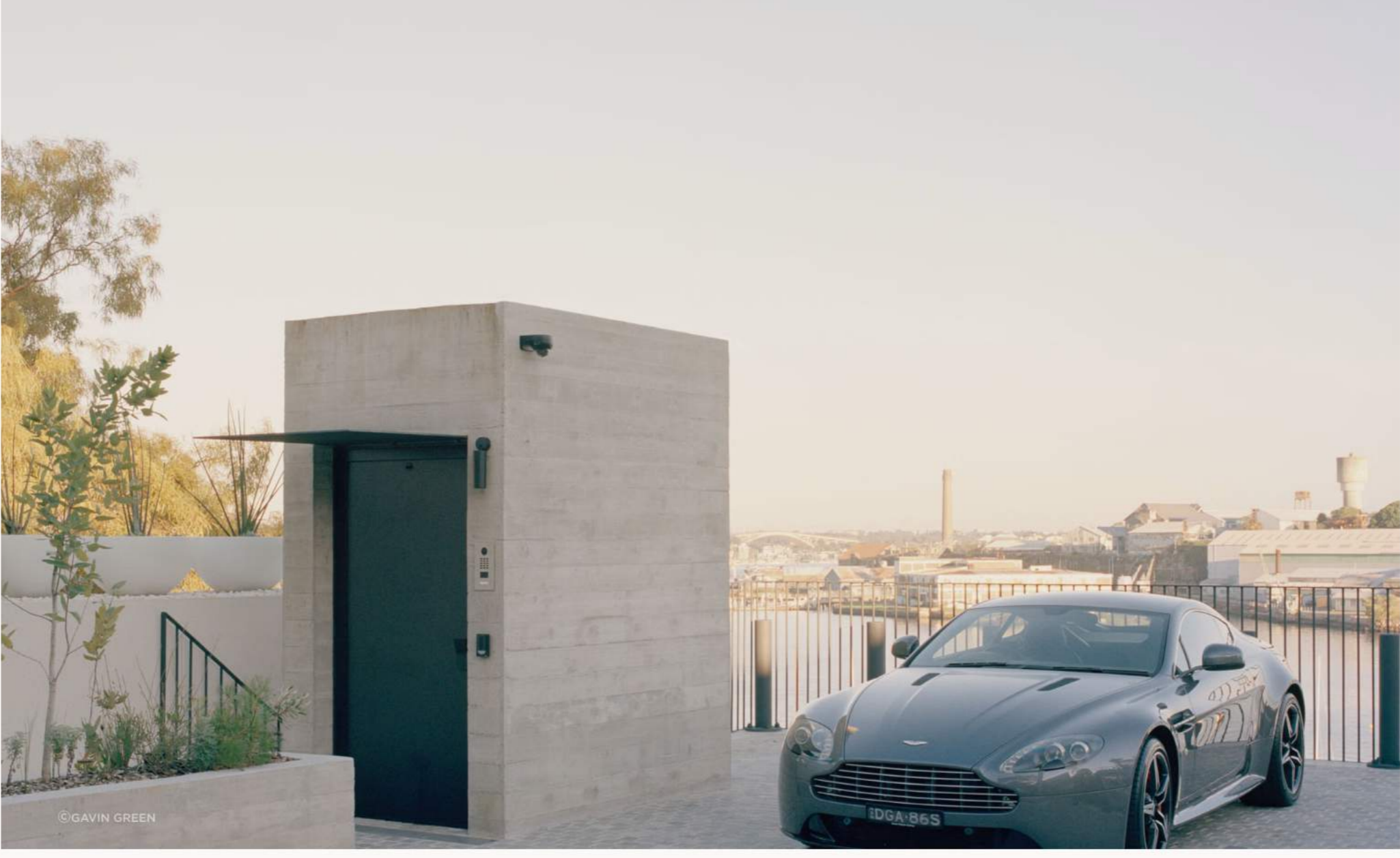
The lift protruding from the concrete form at street level is the only indication of the jaw-dropping structure below.
