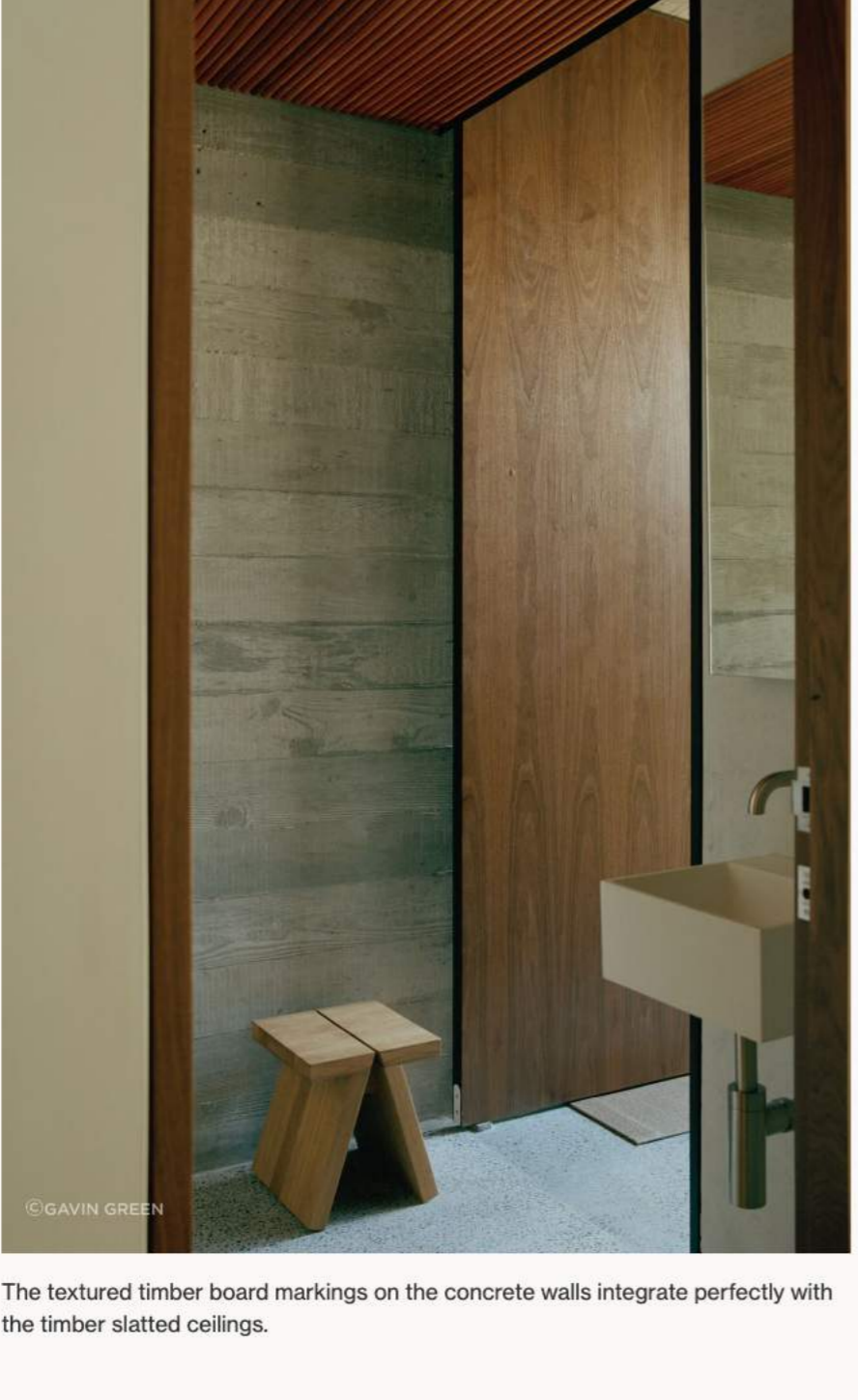
The textured timber board markings on the concrete walls integrate perfectly with the timber slatted ceilings.
