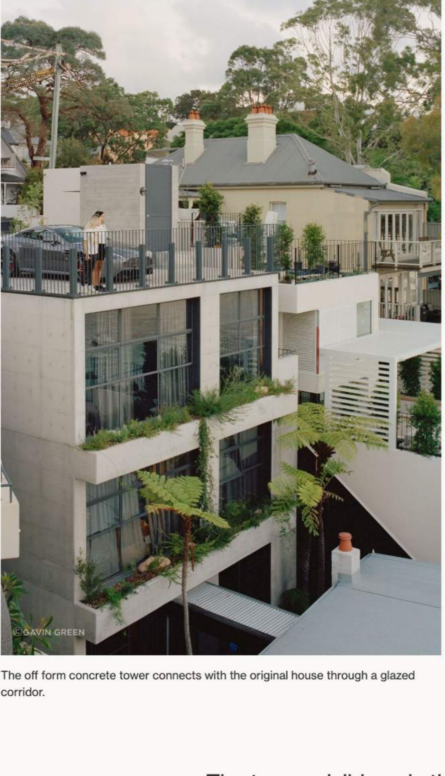
The off form concrete tower connects with the original house through a glazed corridor.
