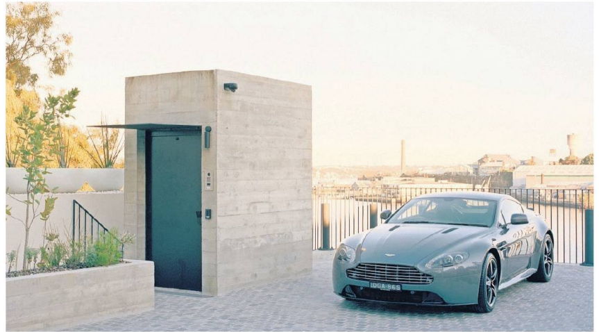
The only sign of a building at street level is a concrete lift shaft.
